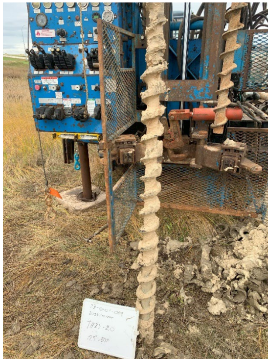
TH23-20 Photo 6: 7.5 m to 8.1 m (25 ft to 27ft)
