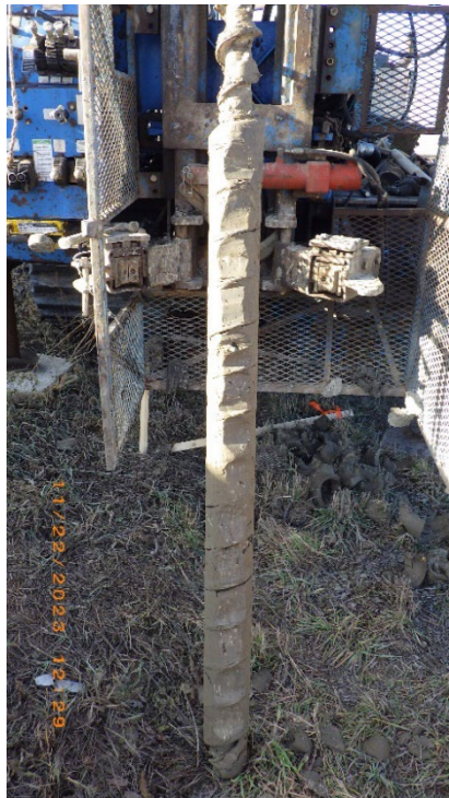
TH23-22 Photo 2: 1.2 m to 2.7 m (4 ft to 9 ft)
