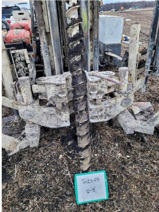
TH23-25 Photo 1: 0.0 m to 1.5 m (0 ft to 5 ft)
