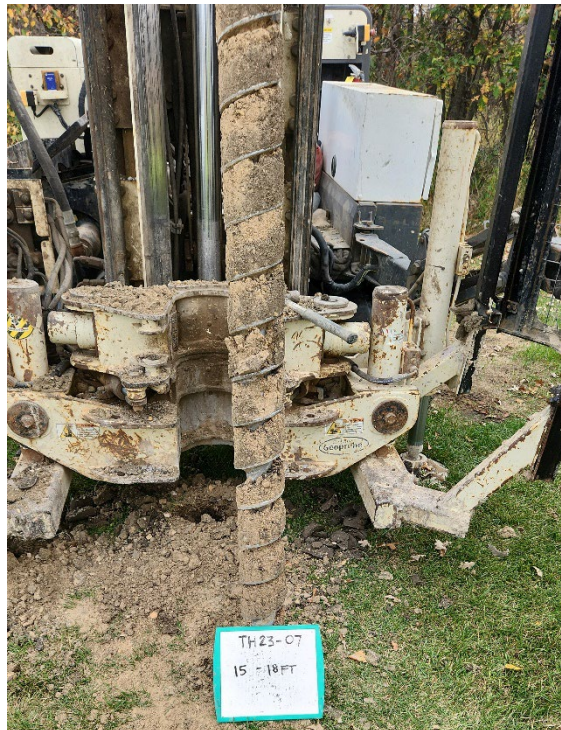
TH23-07 Photo 4: 4.5 m to 5.4 m (15 ft to 18 ft)
