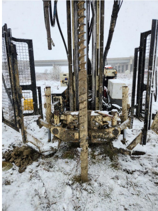
TH23-18 Photo 3: 3.0 m to 4.5 m (10 ft to 15 ft)
