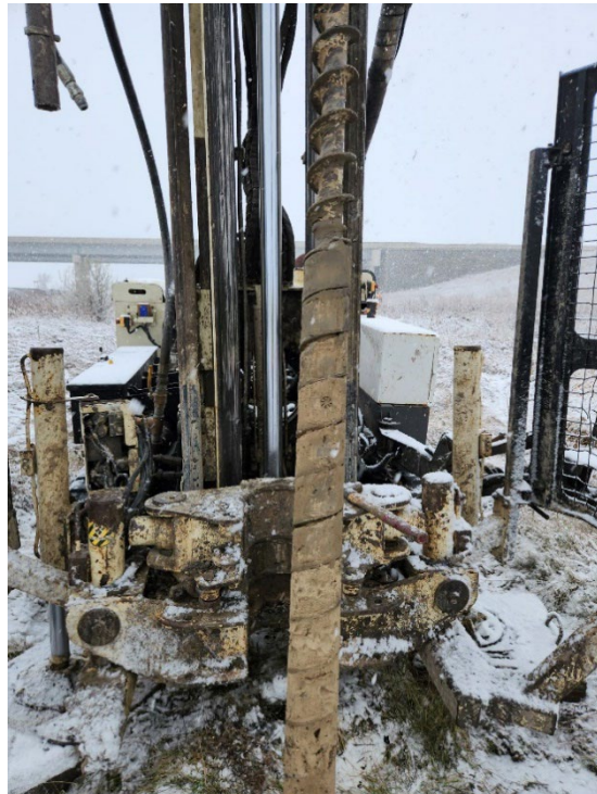
TH23-18 Photo 2: 1.5 m to 3.0 m (5 ft to 10 ft)
