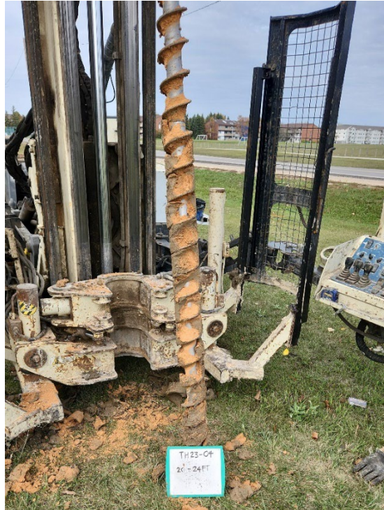
TH23-04 Photo 5: 6.0 m to 7.3 m (20 ft to 24 ft)
