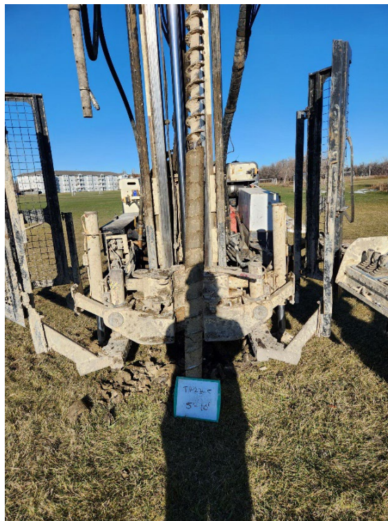
TH23-05 Photo 2: 1.5 m to 3.0 m (5 ft to 10 ft)
