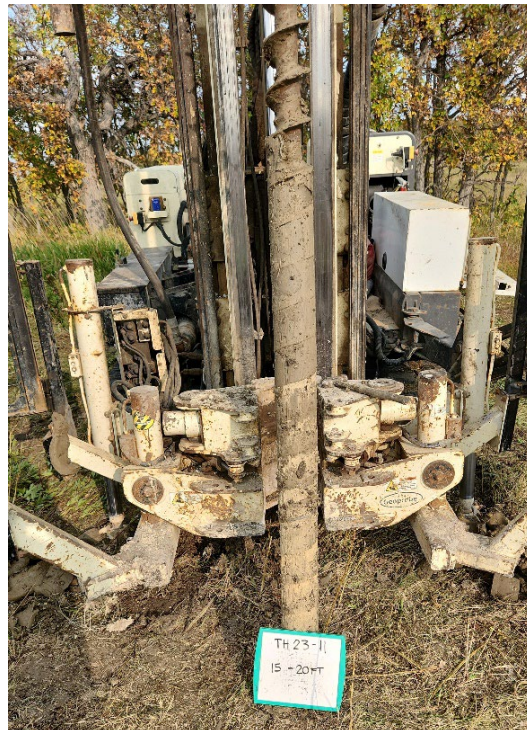
TH23-11 Photo 4: 4.5 m to 6.0 m (15 ft to 20 ft)
