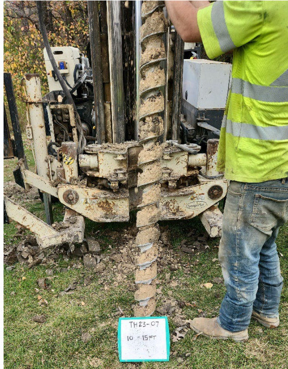
TH23-07 Photo 3: 3.0 m to 4.5 m (10 ft to 15 ft)
