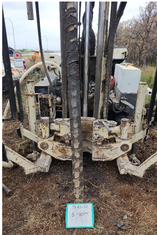
TH23-01 Photo 2: 1.5 m to 3.0 m (5 ft to 10 ft)
