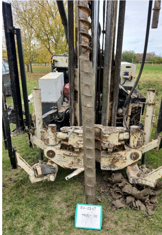
TH23-03 Photo 3: 3.0 m to 4.5 m (10 ft to 15 ft)
