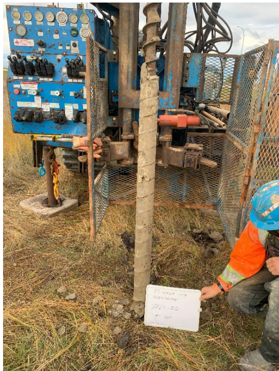
TH23-20 Photo 2: 1.5 m to 3.0 m (5 ft to 10 ft)
