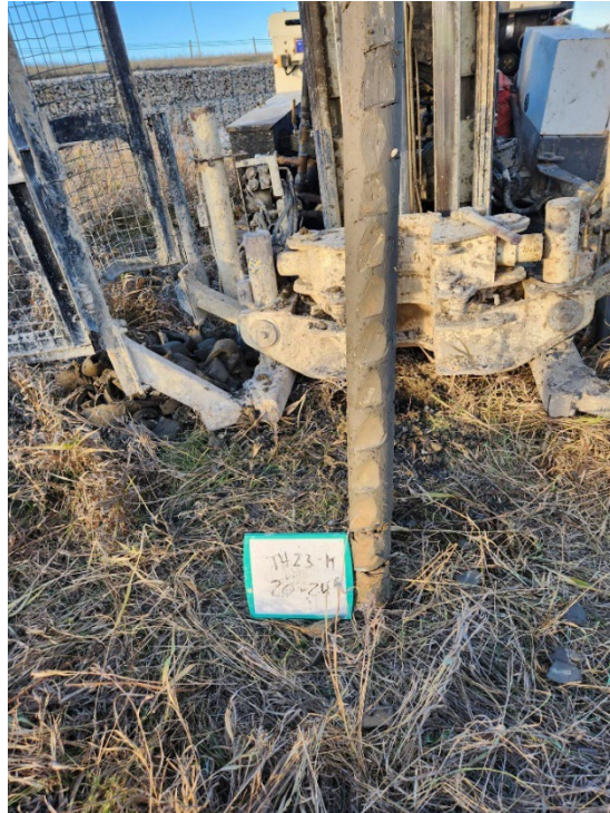
TH23-19 Photo 5: 6.0 m to 7.2 m (20 ft to 24 ft)
