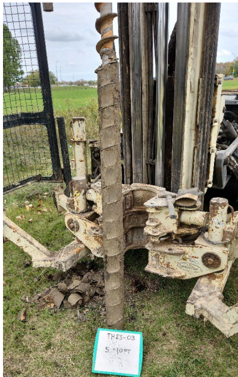
TH23-03 Photo 2: 1.5 m to 3.0 m (5 ft to 10 ft)
