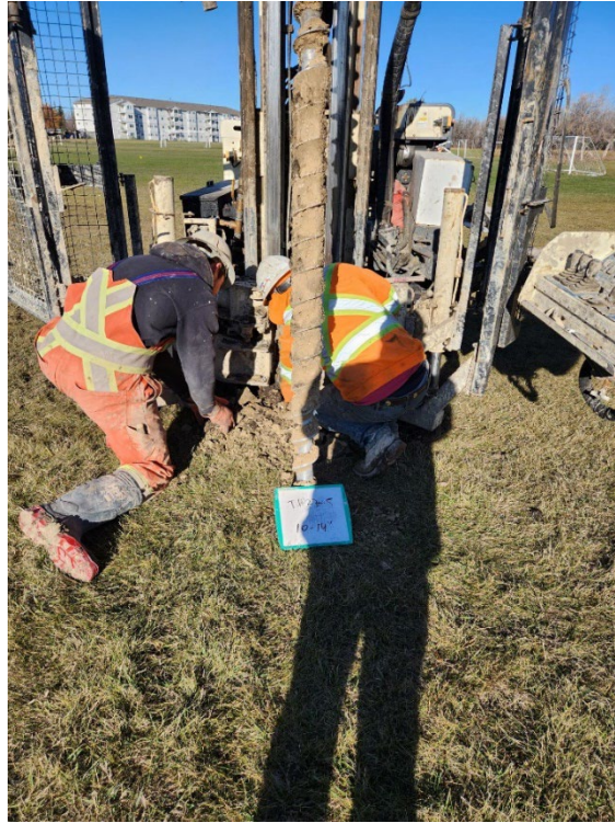
TH23-05 Photo 3: 3.0 m to 4.2 m (10 ft to 14 ft)
