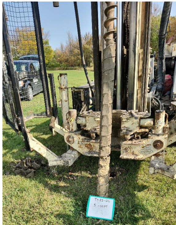
TH23-06 Photo 2: 1.5 m to 3.0 m (5 ft to 10 ft)
