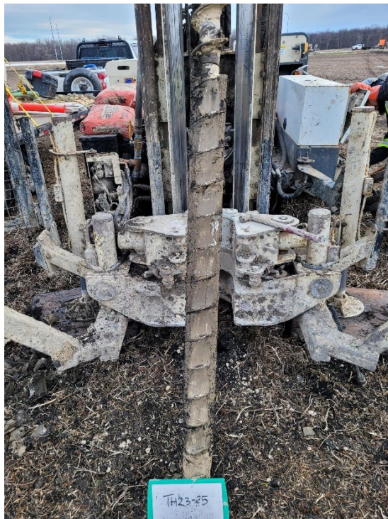
TH23-25 Photo 2: 1.5 m to 3.0 m (5 ft to 10 ft)
