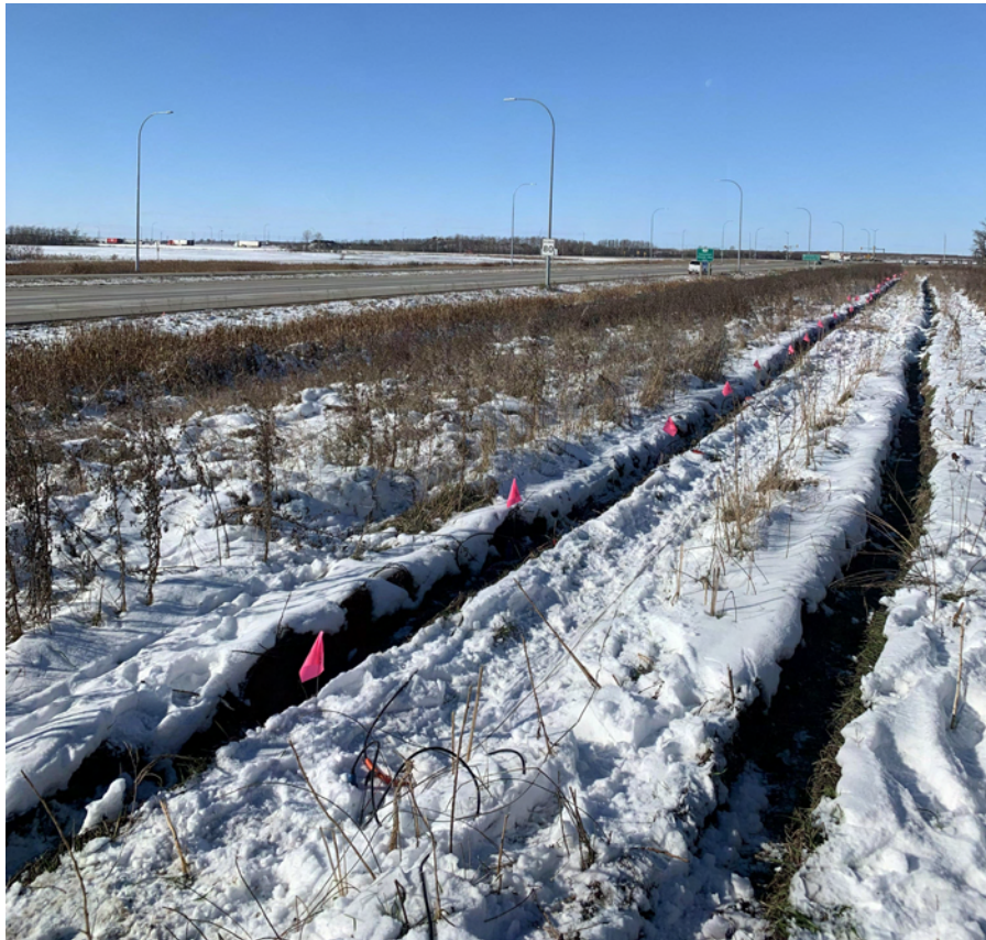
Line SL23-03 Looking Northwest
