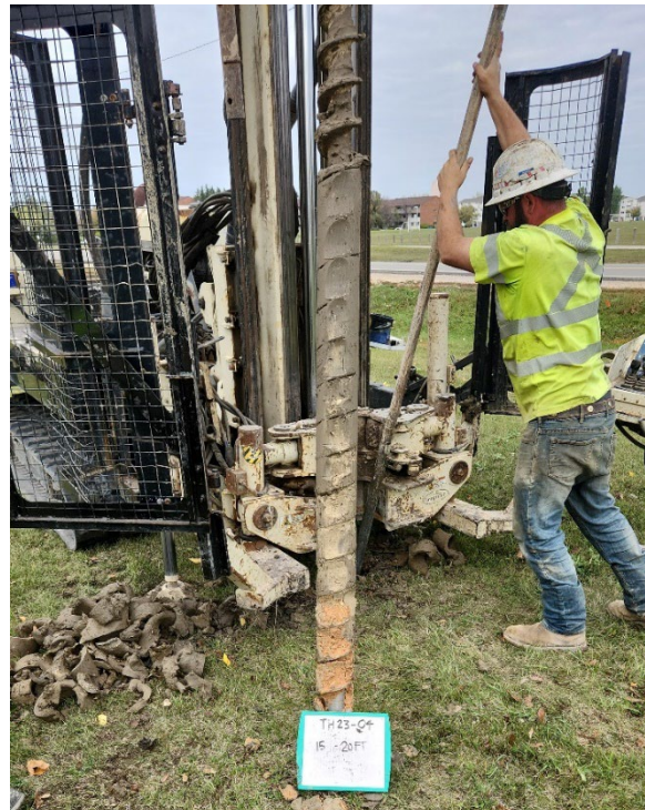
TH23-04 Photo 4: 4.5 m to 6.0 m (15 ft to 20 ft)
