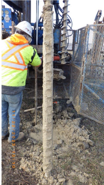
TH23-22 Photo 7: 5.7 m to 7.2 m (19 ft to 24 ft)
