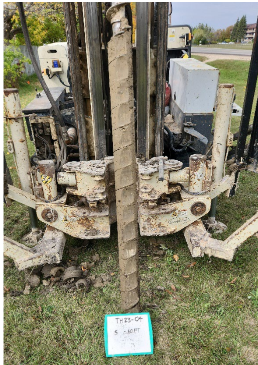
TH23-04 Photo 2: 1.5 m to 3.0 m (5 ft to 10 ft)
