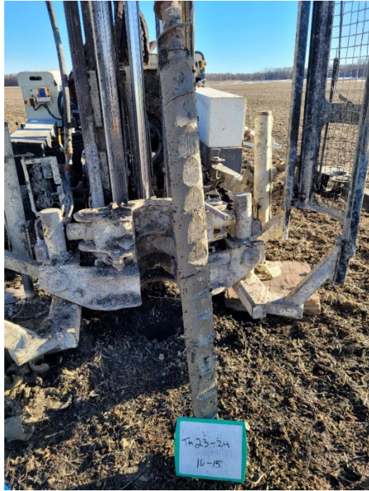
TH23-24 Photo 3: 3.0 m to 4.5 m (10 ft to 15 ft)
