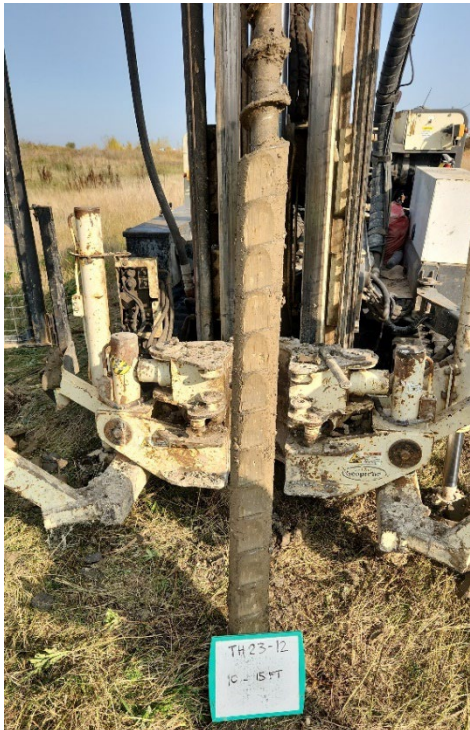
TH23-12 Photo 2: 3.0 m to 4.5 m (10 ft to 15 ft)
