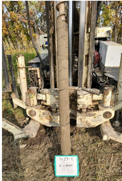
TH23-11 Photo 2: 1.5 m to 3.0 m (5 ft to 10 ft)
