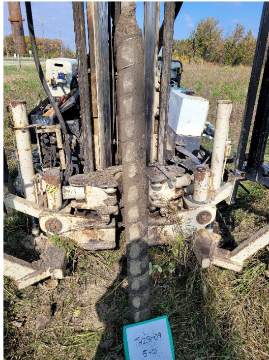
TH23-09 Photo 2: 1.5 m to 3.0 m (5 ft to 10 ft)
