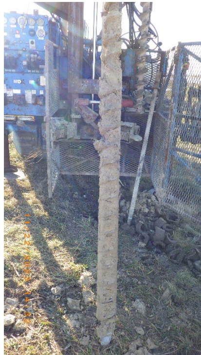
TH23-21 Photo 6: 5.7m to 7.2 m (19 ft to 24 ft)
