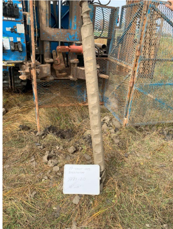
TH23-20 Photo 3: 3.0 m to 4.5 m (10 ft to 15 ft)
