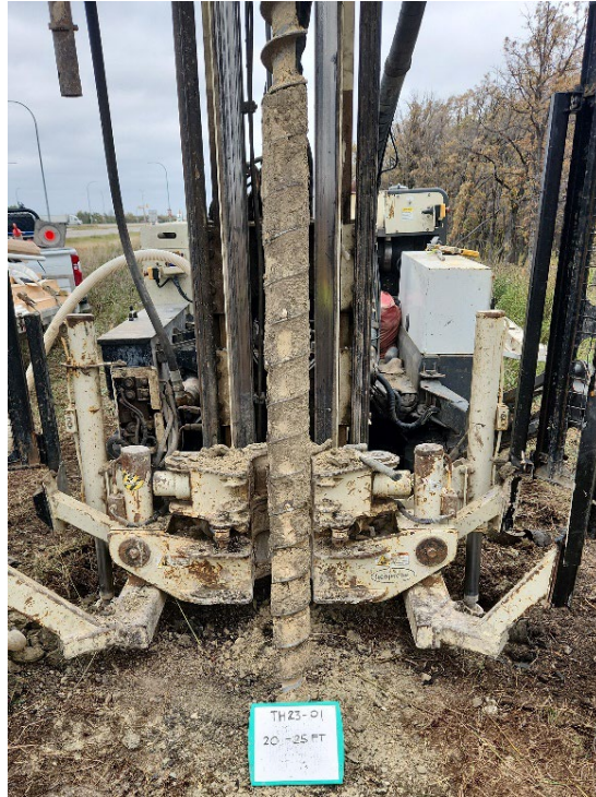
TH23-01 Photo 5: 6.0 m to 7.5 m (20 ft to 25 ft)
