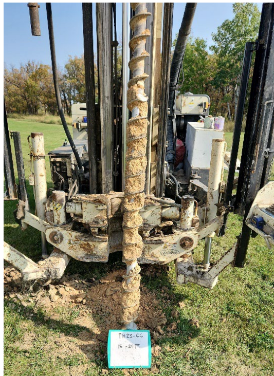
TH23-06 Photo 4: 3.0 m to 4.5 m (15 ft to 20 ft)
