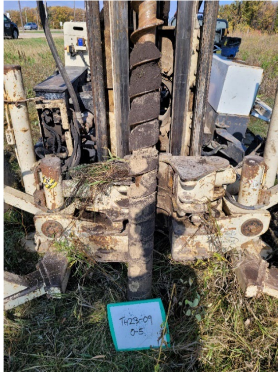
TH23-09 Photo 1: 0.0 m to 1.5 m (0 ft to 5 ft)
