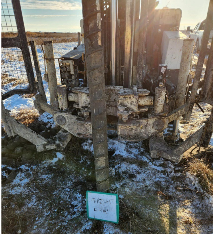
TH23-17 Photo 3: 3.0 m to 4.2 m (10 ft to 14 ft)
