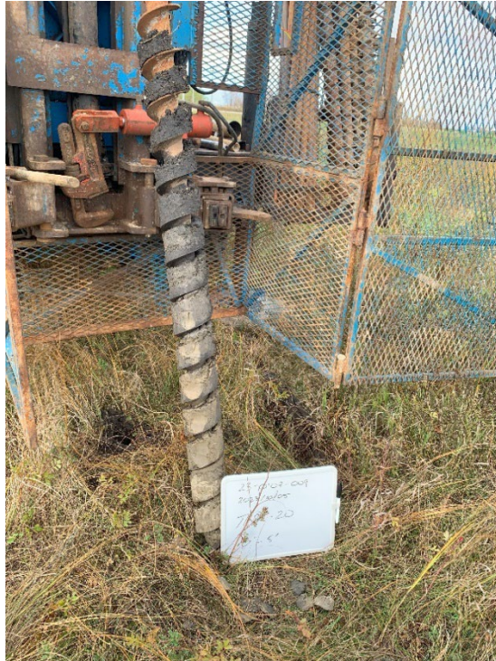
TH23-20 Photo 1: 0.0 m to 1.5 m (0 ft to 5 ft)
