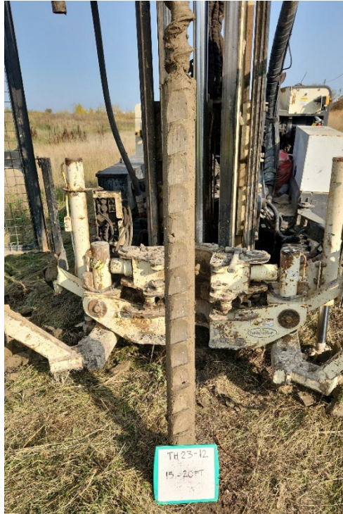
TH23-12 Photo 3: 4.5 m to 6.0 m (15 ft to 20 ft)
