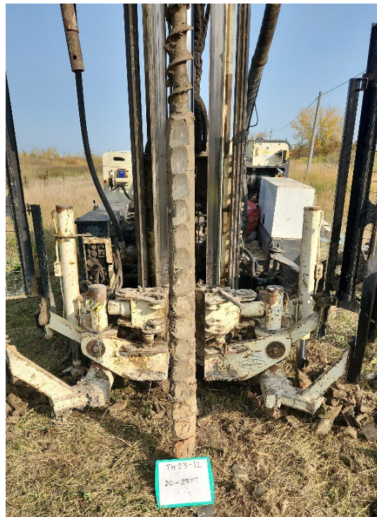
TH23-12 Photo 4: 6.0 m to 7.5 m (20 ft to 25 ft)
